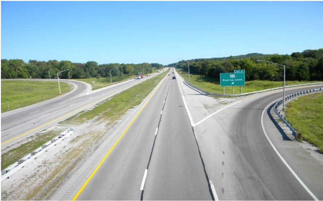
Photo 1: On WN 9007 at US 231 ramp facing North.
