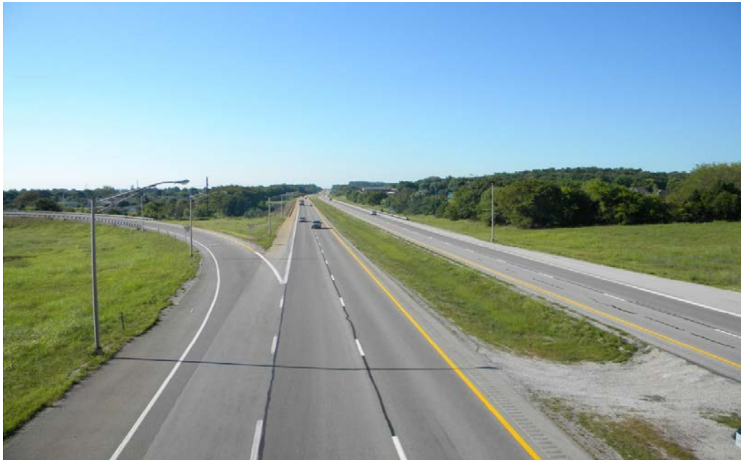
Photo 2: On WN 9007 at US 231 ramp facing South.
